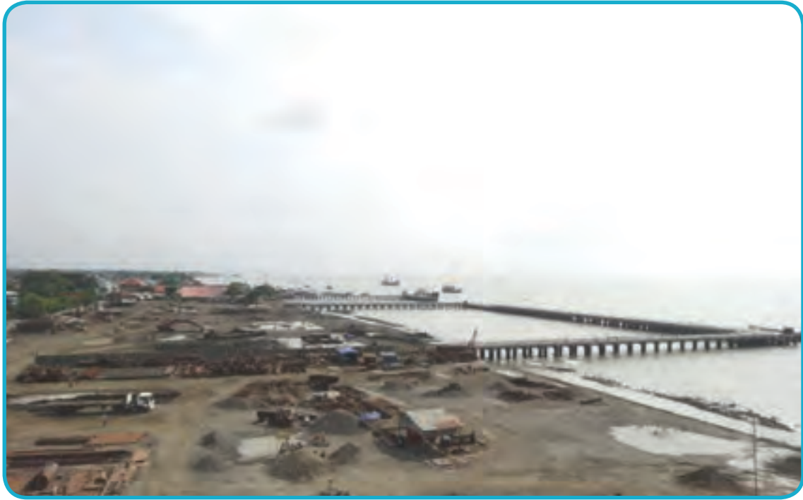
The Sittwe port with the Port and IWT Jetty already constructed
