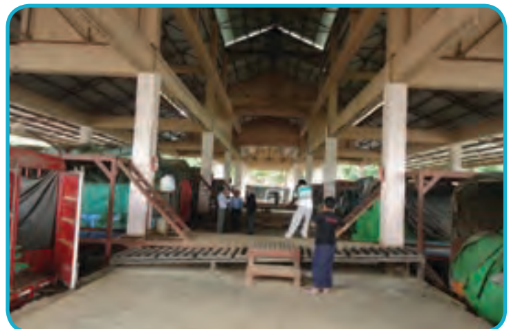
Export Inspection Platform. Twelve trucks can be parked on either side
