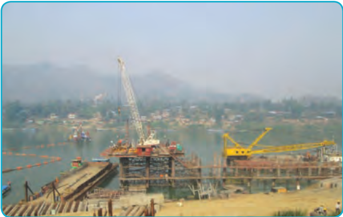
Construction work on IWT terminal in progress at Paletwa
