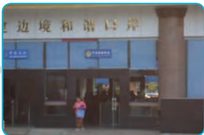
Close up shot of middle gate. Left side.
