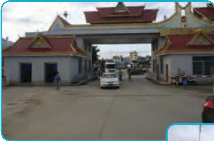
Full view of third gate. A large truck waiting at the left gate on China side.
