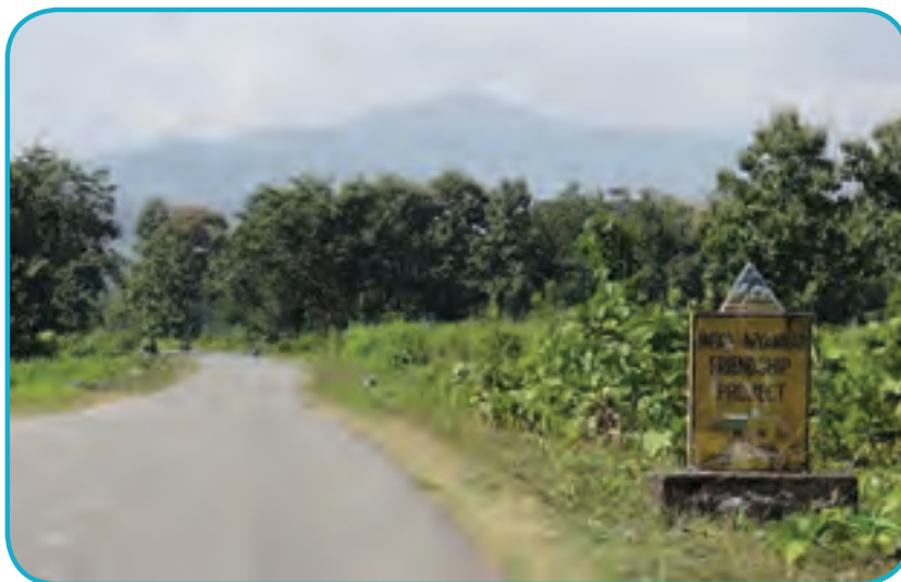
Tamu-Kalewa Road after resurfacing
