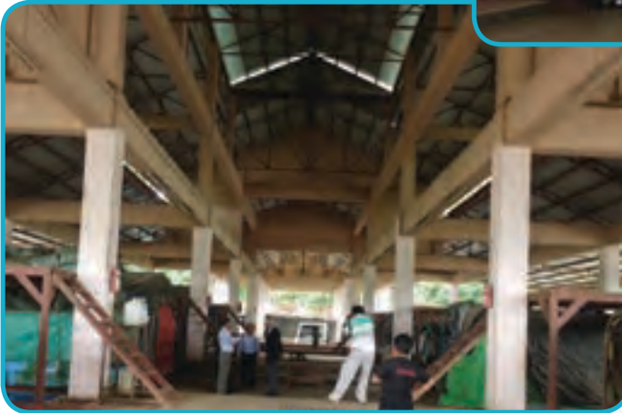
Export Inspection Platform. Twelve trucks can be parked on either side
