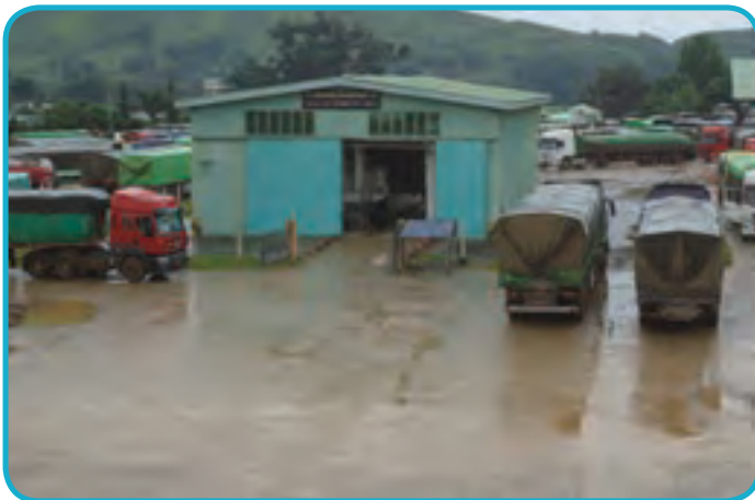
The building housing the X-ray facility at the 105 mile Trade Zone
