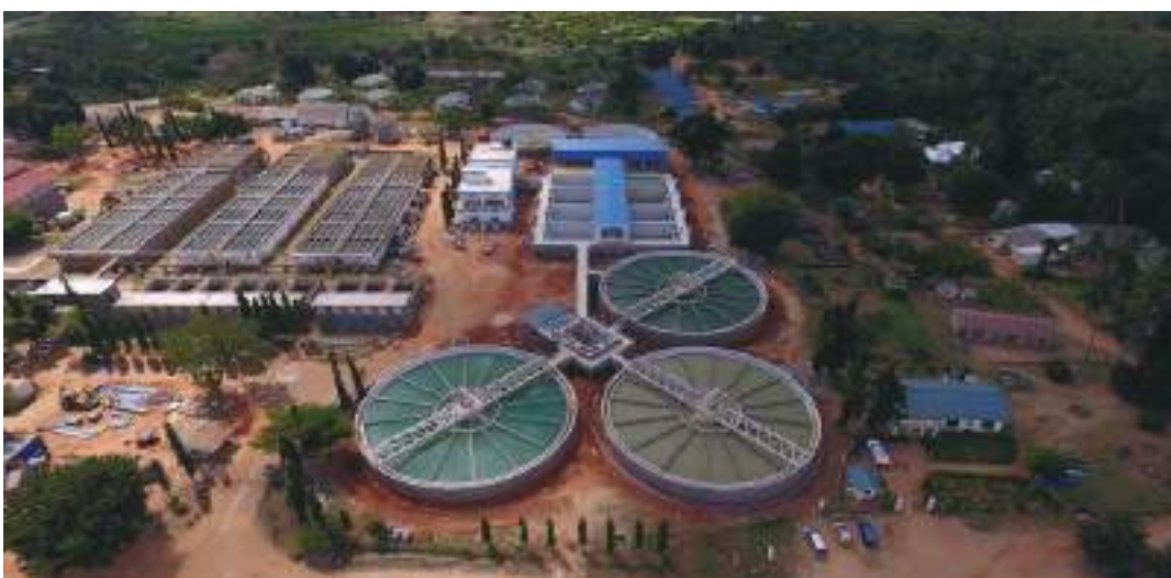
Part of Ruvu Water Project
